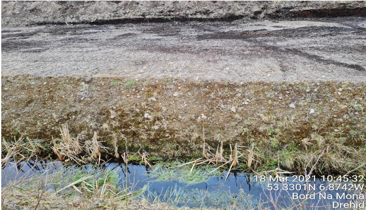
Plate 1-1: Exposed subsoils beneath stripped peat near the landfill expansion area
